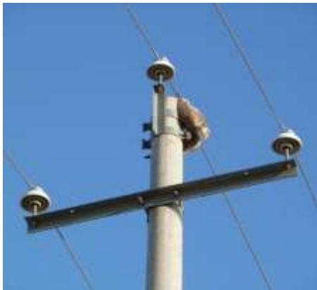
Image 3,4: Pylon with centre top pins and dead Saker, Mongolia (photo: A. Dixon) and retrofitted, safe for birds (photo O. Dorjsuren)
