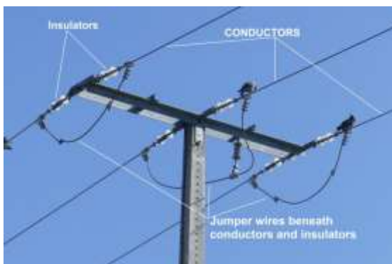
Image 2: Example of proper design of strain insulators (it is the same configuration to deadend insulators) (photo J. Martin Martin & A. Camiña)
