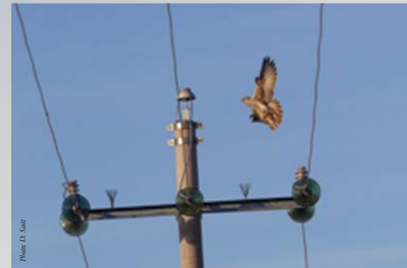
Saker about to land on power pole in Mongolia with inappropriately deployed perch deflector spikes, which increase the risk of electrocution
